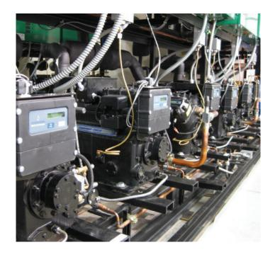
The rack was operating with 900 compressor cycles per day. We were days away from our grand opening, and tried a variety of controlling methods to reduce cycle counts and still maintain product temperatures without success. We retrofitted the digital unloader on only one compressor and the impact was amazing. Within minutes of activation, compressor cycles were reduced to 12 starts in four days for the entire rack.
