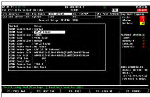
Figure 10-19 - I/O Network Baud Rate Setup
