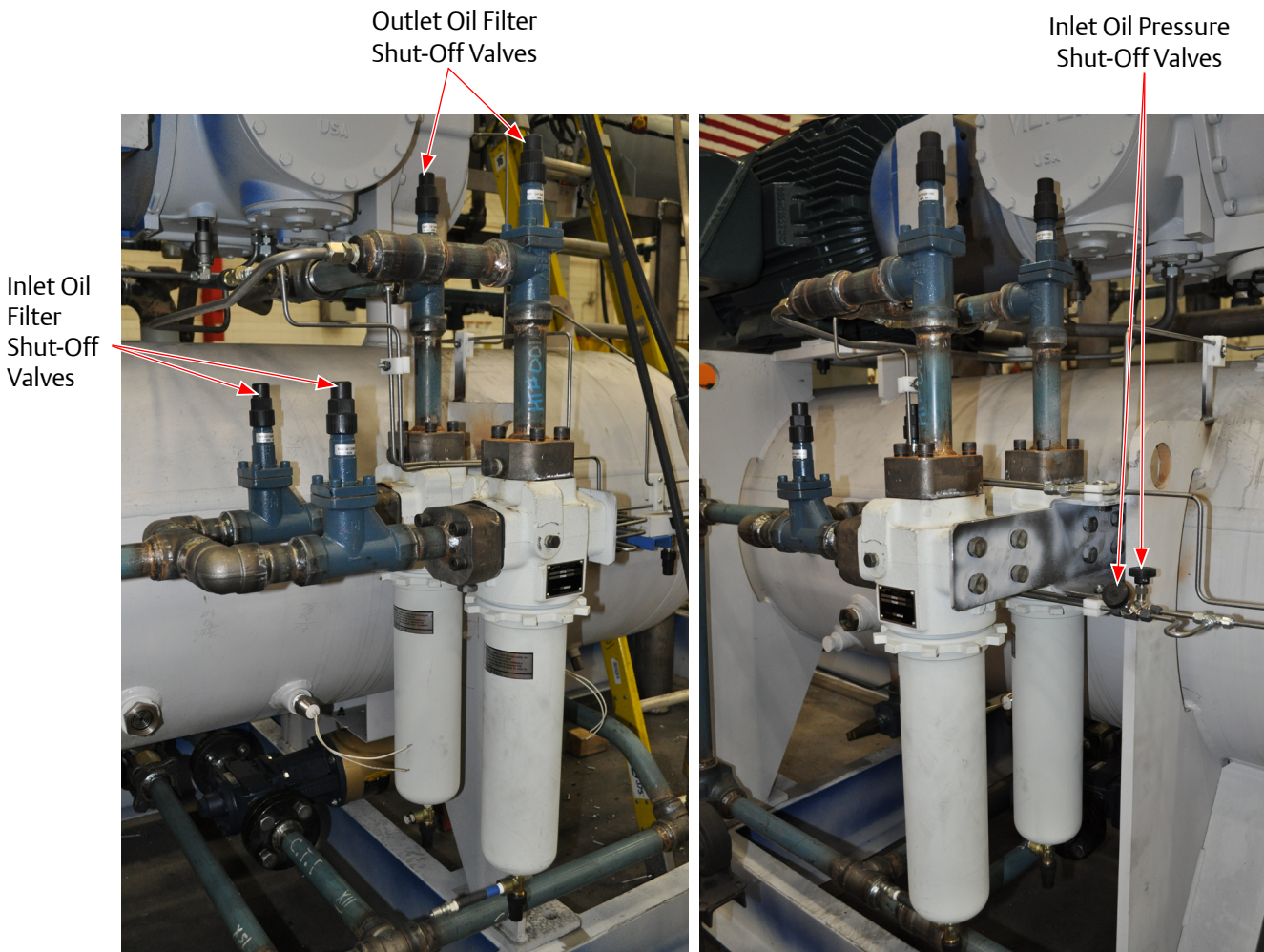
Figure 4-15. Dual Oil Filter Setup for Oil Filters with Manifold Heads
