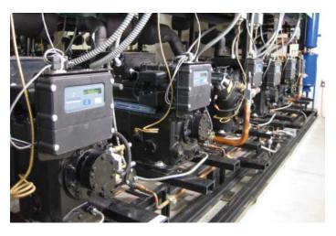
By integrating several traditional components into one control module, the Copeland Discus Digital compressor with CoreSense Diagnostics modules requires less wiring and fewer connection points, improving system quality and ensuring installation ease and consistency.
