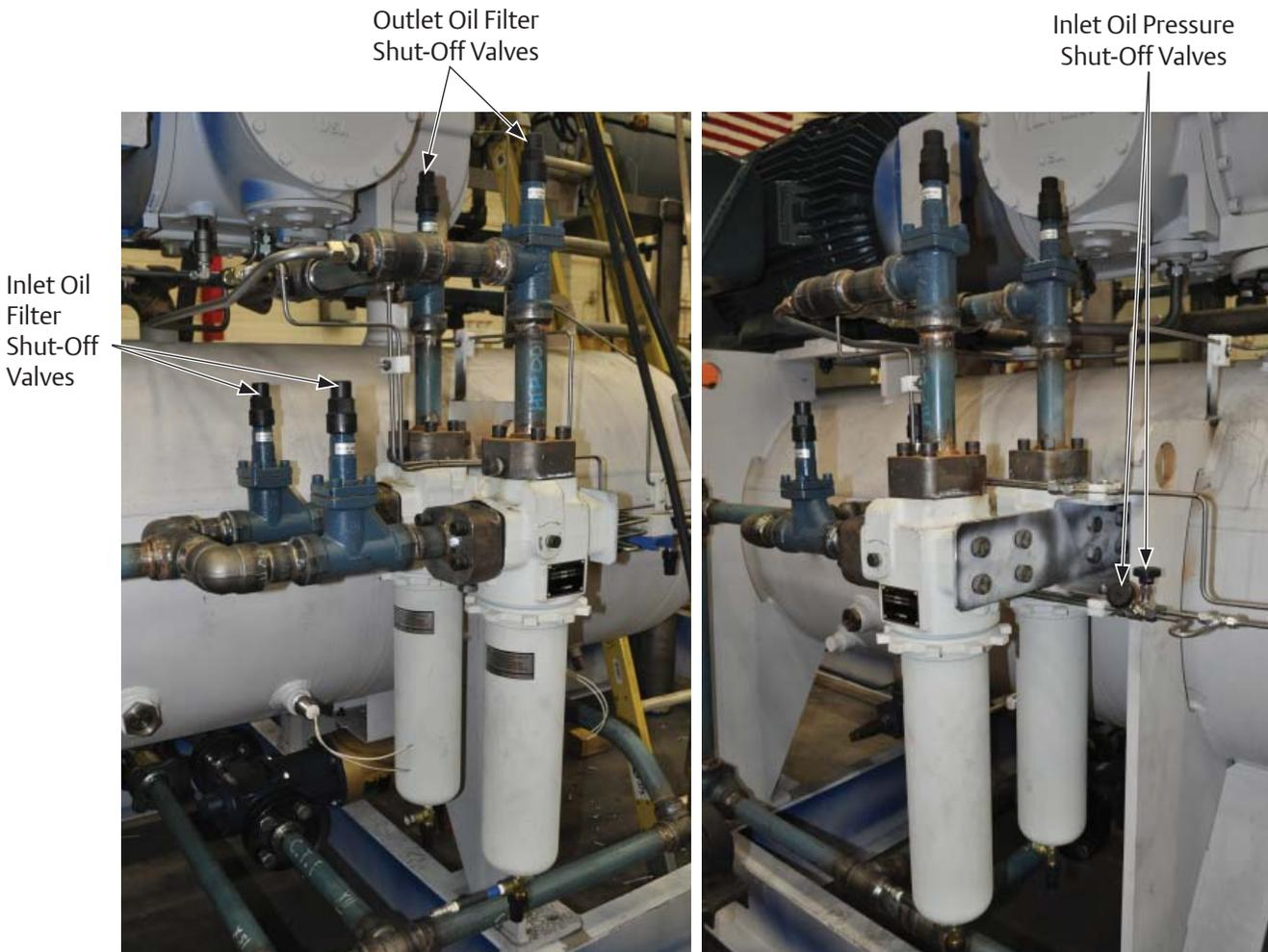
Figure 4-9. Dual Oil Filter Setup for Oil Filters with Manifold Heads
