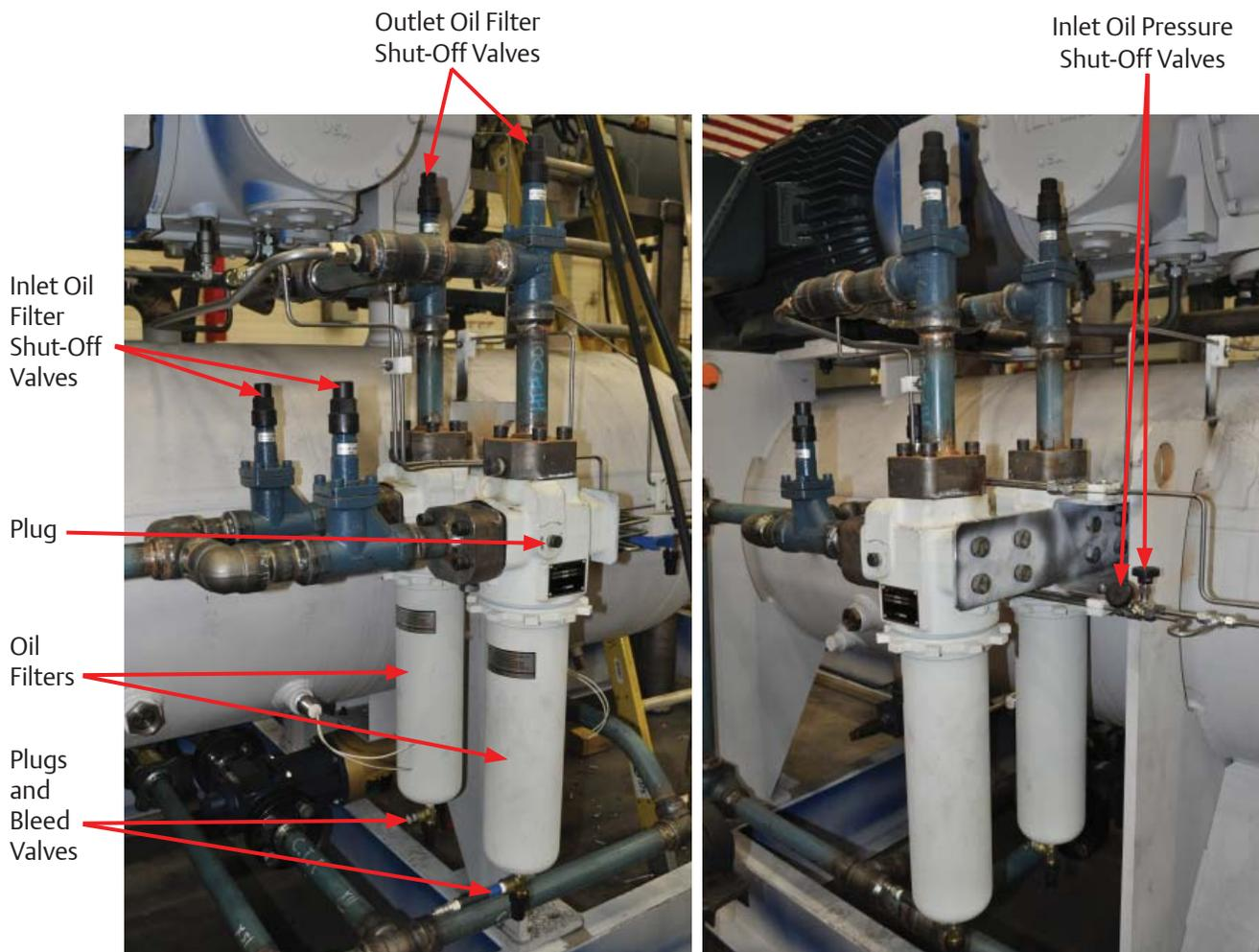
Figure 5-8. Dual Oil Filter (3111A Oil Filter Housings Shown)
