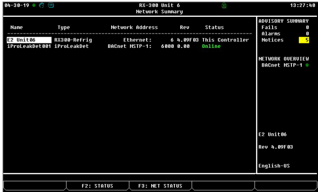
Resetting Spill Alarm Network Summary Screen
