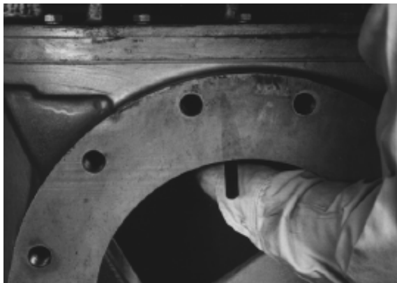
FIGURE 7-19 – DISCHARGE END CLEARANCE CHECK
