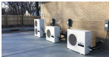
Ultra-quiet variable speed fan motors and internal baffling further improve the sound quality, creating a better customer experience and providing additional location options.
