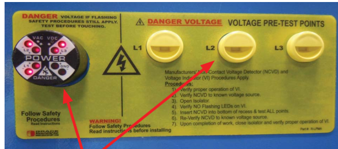
Redundant Voltage Verification – Visual Indicator and Non-Contact Voltage Portal
