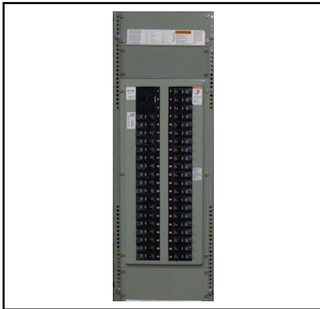
Figure 1-1 - Eaton Panel Breaker
