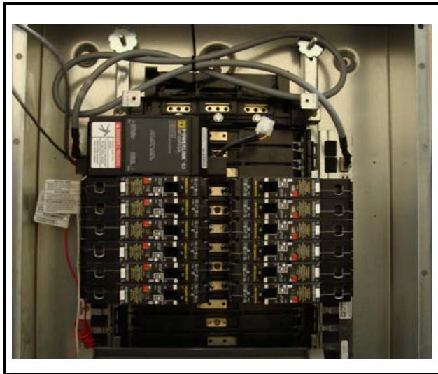
Figure 1-2 - Square D Powerlink Breaker Panel (24-Breaker Version Pictured)
