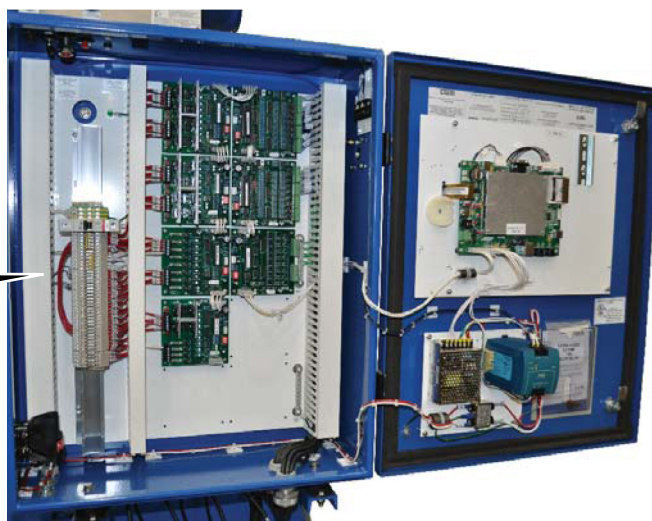
Figure 4-5. Wire Connections for Capacity and Volume Actuators
