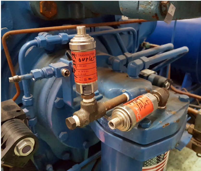
Figure 5. Tri-Micro filter with pressure transducers
