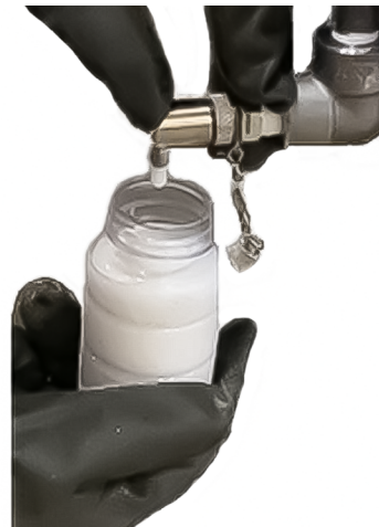
Figure 5-5. Operating the Oil Sampling Valve
