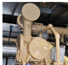
Single screw compressor with suction strainer & check valve
