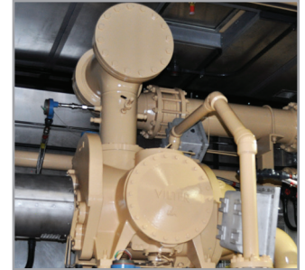
Single Screw Compressor with Suction Strainer & Check Valve
