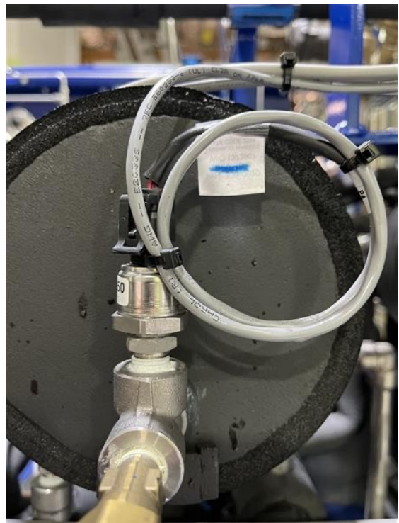
Figure 3 - Transducer Cable Harness
