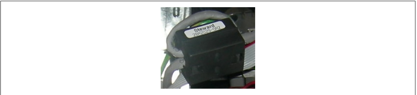
Figure 3 - Ferrite Installation of Ethernet Cable
