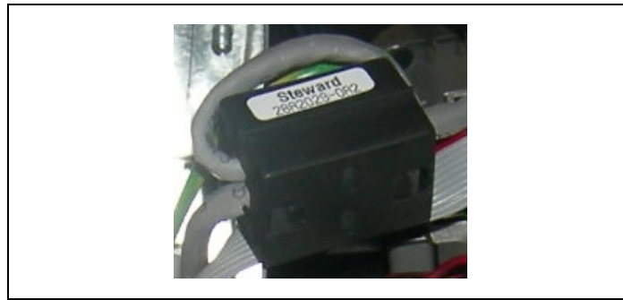
Figure 3 - Ferrite Installation of Ethernet Cable
