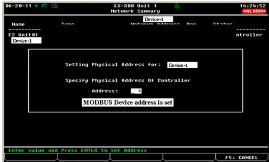
Figure 8 - MODBUS Address Setting
