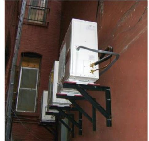
Manhattan Diner, located in NYC at 94th & Broadway, could not install conventional condensing units on the roof of its six-story building due to space constraints. A seven-foot wide alley was the only other location option. The X-Line condensing unit's **slim profile allowed the units to be installed safely on the building** wall using heavy-duty brackets – high enough not to interfere with the ground areas between New York City's alleyways.
